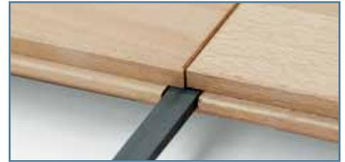
Lengthwise the panels have a tongue and groove connection and at ends the panels are joined using loose tongues.
