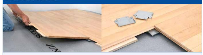
Each floor panel is easily locked into position with the pre-mounted metal joining brackets.
